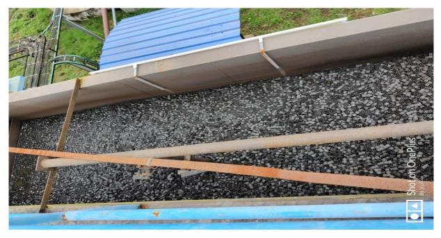
Fig. 18.17 Moving Bed Bio Reactor in the Septage treatment plant, Willingdon island
