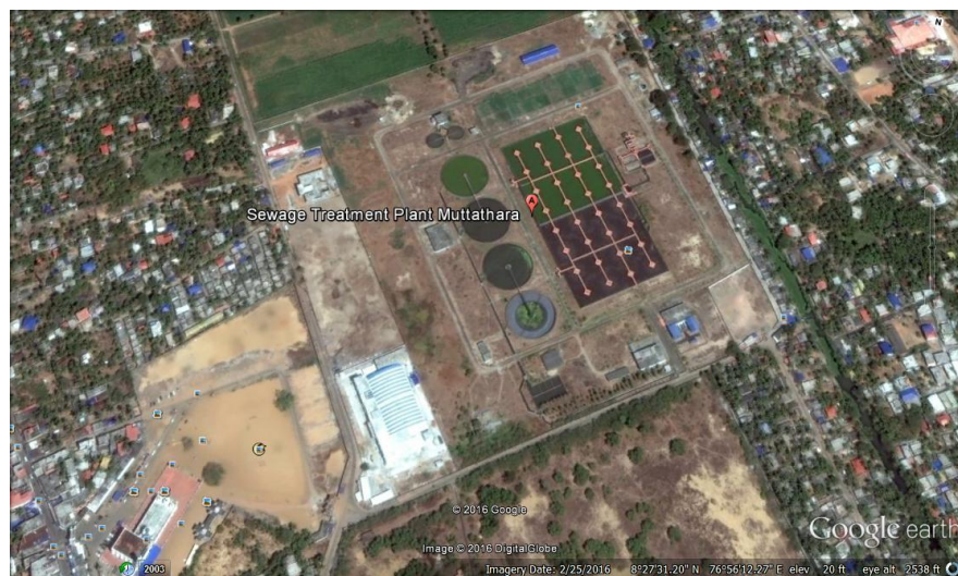
Fig. 18.27 Location of Muttathara sewage treatment plant
