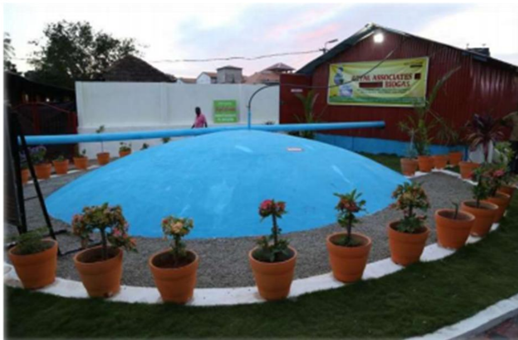
Figure 18.3 Community Level Biogas plant
