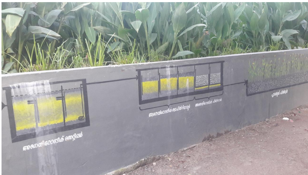
Fig.18.20 Planted gravel filter in DEWATS system in the slum area at Chathanad
