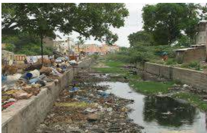
Figure 6.1: Indiscriminate dumping of C & D waste results in choking drains
