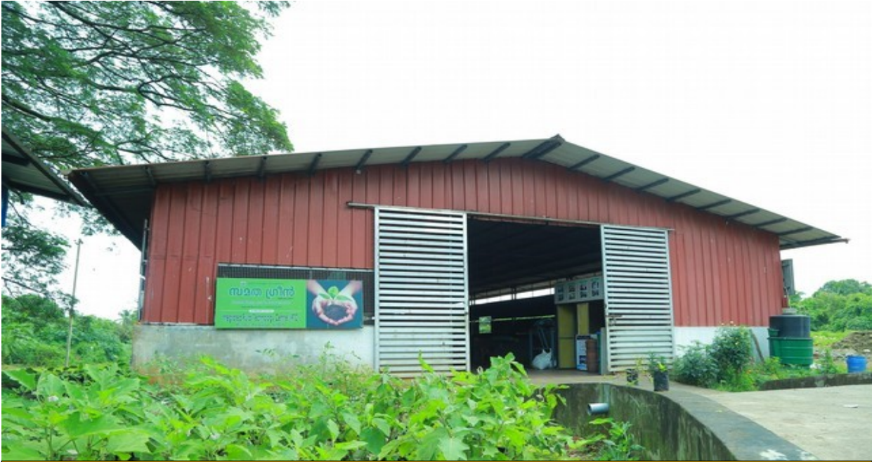
Green Park, Kurukkanpara, Kunnamkulam Municipality (Solid waste management plant) operated and maintained by SHG, Samatha Green
