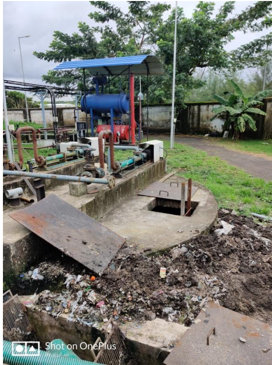
Fig.18.18 Septage collection tank
