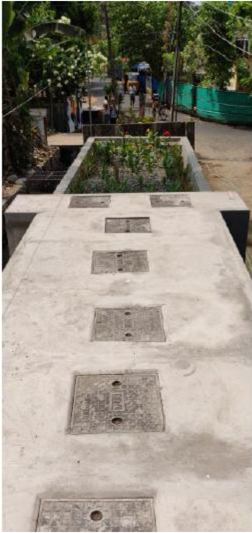
Fig.19.22 The anaerobic baffled reactor
