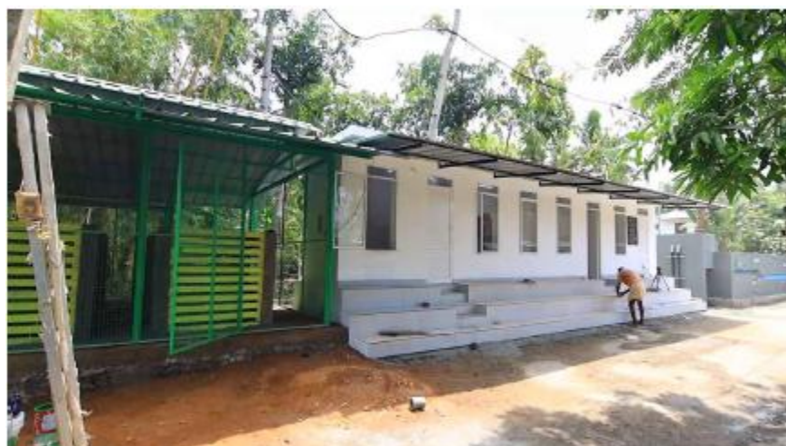
Fig.18.26 The newly constructed aerobic unit and the refurbished public toilet
