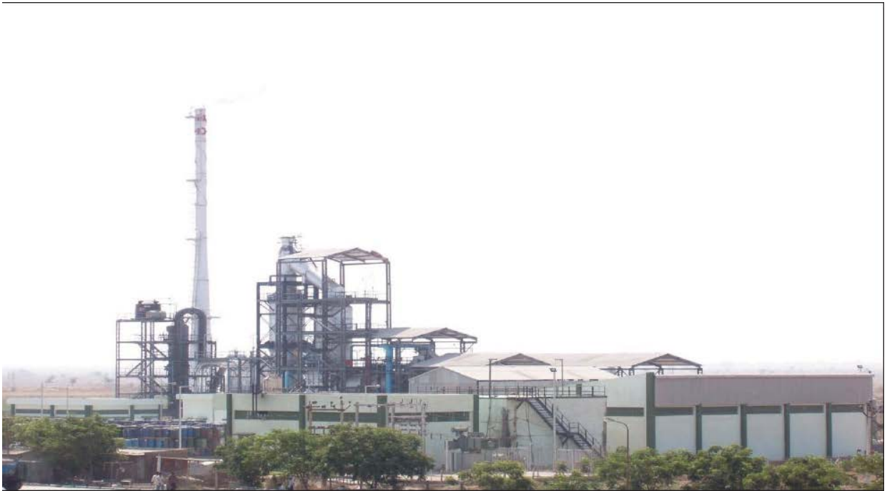
Figure 6.2: Common Hazardous Waste Incinerator at Ankleshwar, Gujarat
