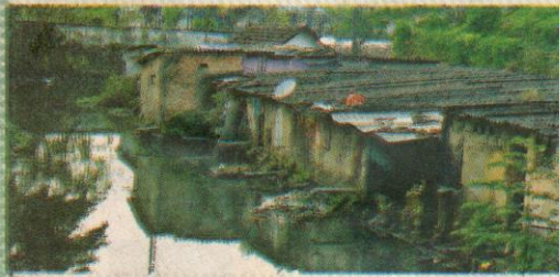
Sewage pipes from houses situated on the banks of Perandoor canal drain but into the water body, resulting in massive pollution | A SANESH
