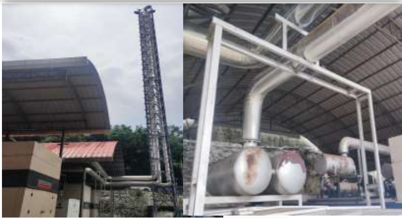
WOOD FIRED BOILER WITH CHIMNEY
