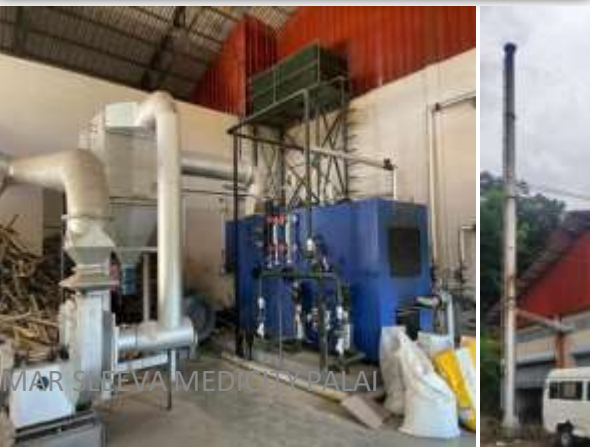
WOOD FIRED BOILER WITH CHIMNEY
