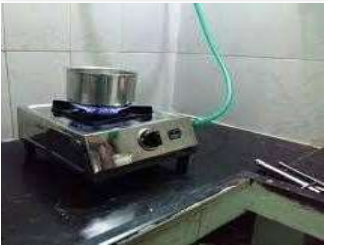
UTILIZATION OF STP GAS FOR COOKING
